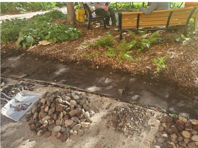
Part of the main swale emptied
