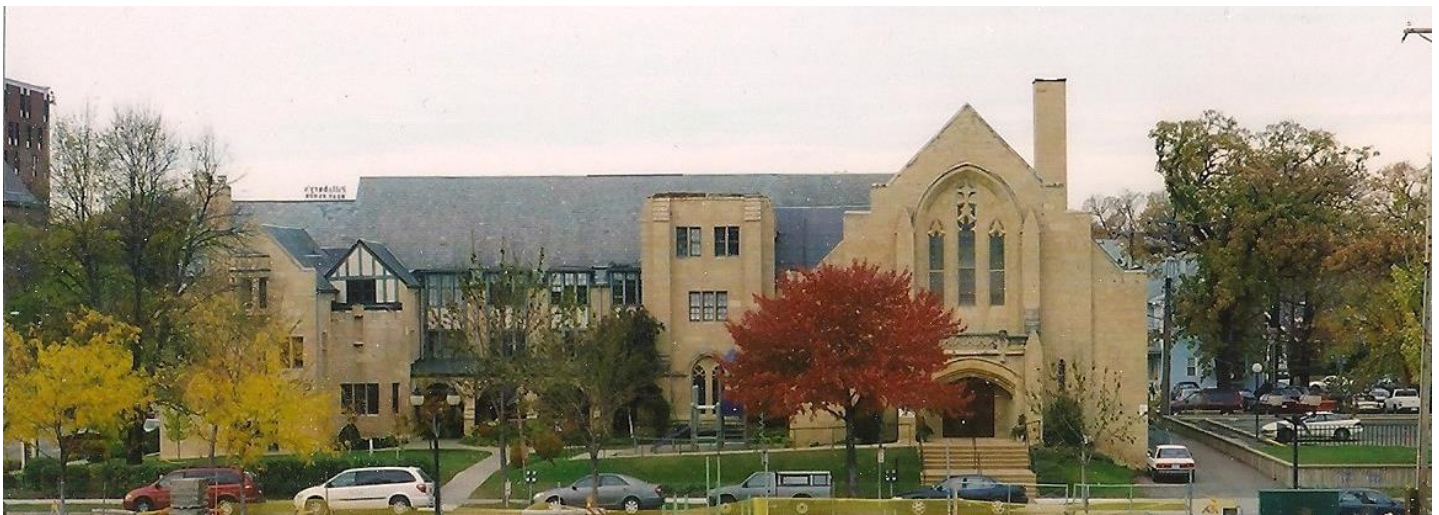
Photo of UBC (year unknown) taken from the roof of Annie's Parlour and before the new apartment building across the street from UBC, was completed. Photo by Don Follett
